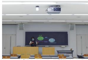
Lecture room setup: The blackboard is captured by an AW-HE40HW installed on the ceiling
